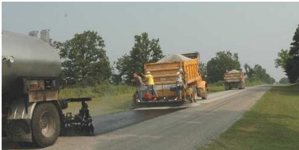
County road crews refinish chip and seal roads.
